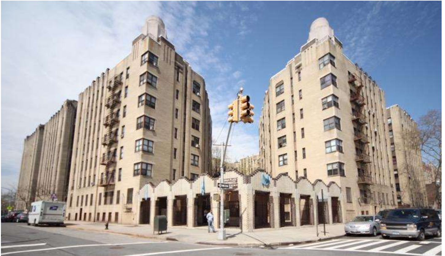
Figure 3. Noonan Plaza Apartments complex, seen from the main entrance at the intersection of 168th Street and Nelson Avenue. Source: Provided by Danois Architects, P.C., taken from the New York Landmarks Preservation Commission (LPC) designation dossier (2010).
